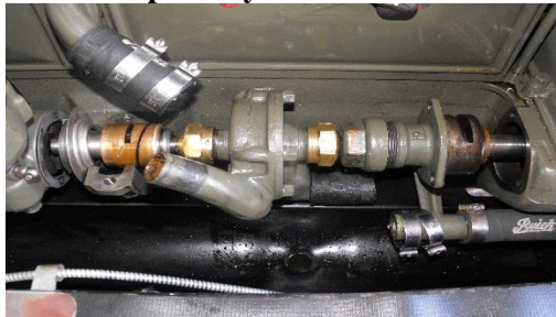
Pump ready for removal
