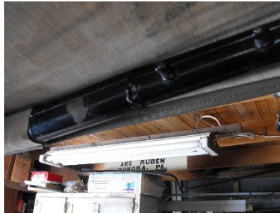
Cut out and re-welded section.
